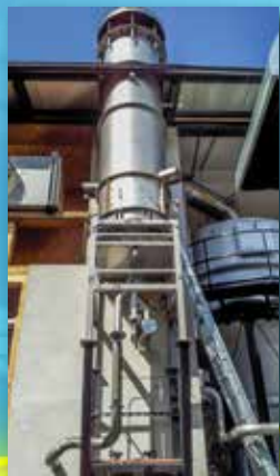
← Wood gas flare for 700 m 3 /h wood gas in Italy
