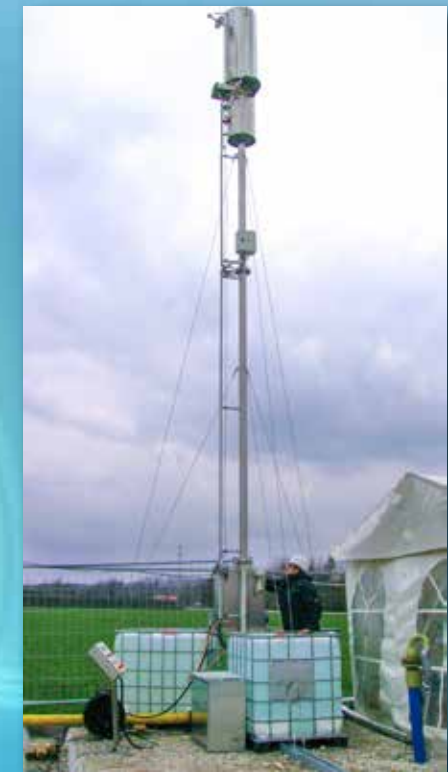
Foldaway wood gas flare for geothermic bore ↑ Germany
